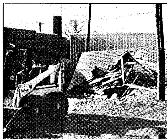
1985 — Construction of current building begins
